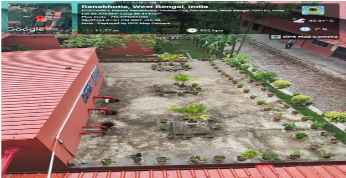
[C]: Reservoir /storage ( 12.5 m X 10 m X 1.6 m)
